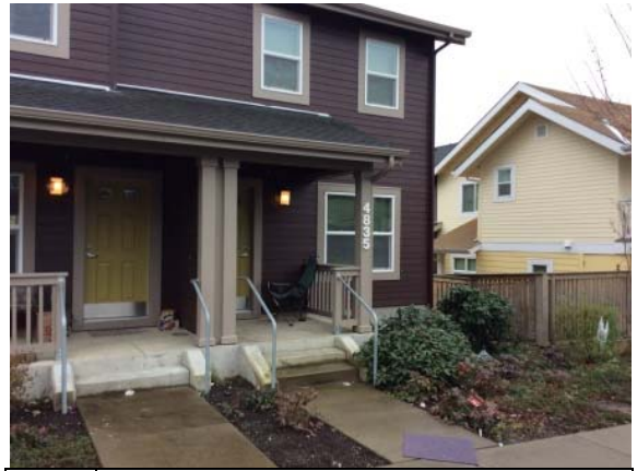
Photo #14: Apartment front entrance with handrails and concrete steps
