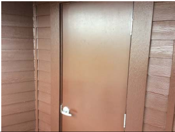
Photo #15: Second floor apartment exterior storage closet
