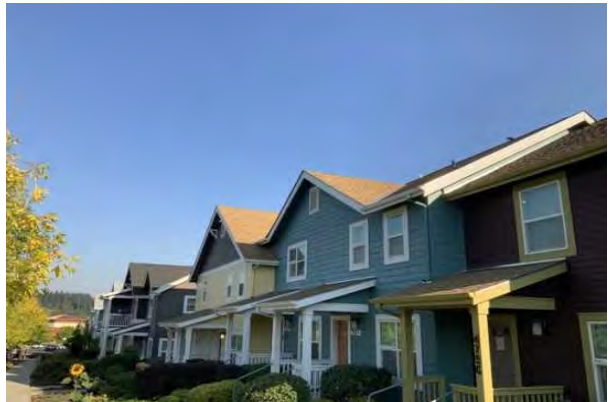
4 ASPHALT SHINGLE ROOF
