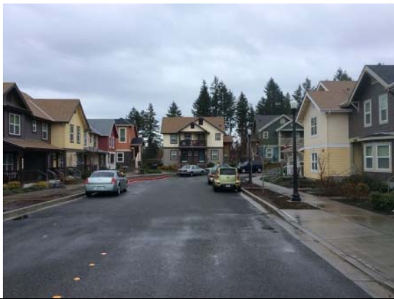
Photo #3: Apartment front elevation
