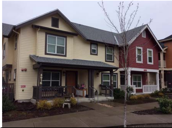
Photo #2: Apartment front elevation
