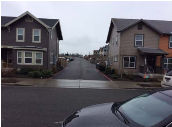
Photo #9: Parking area and driveway between apartment buildings
