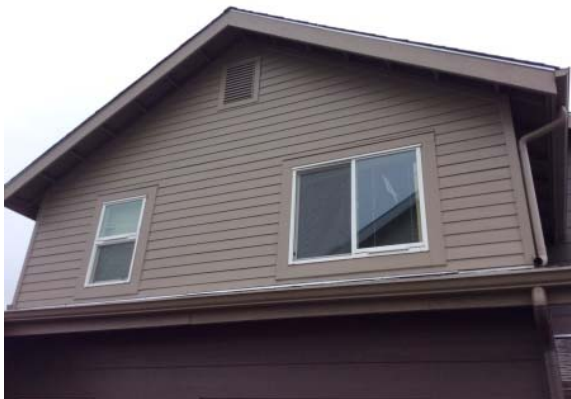
Photo #7: Siding with attic gable vent
