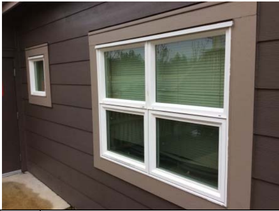
Photo #13: Vinyl framed window
