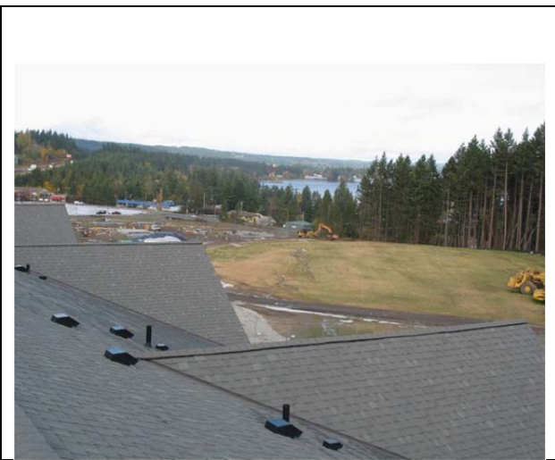
Looking NW at future Bay Vista West
