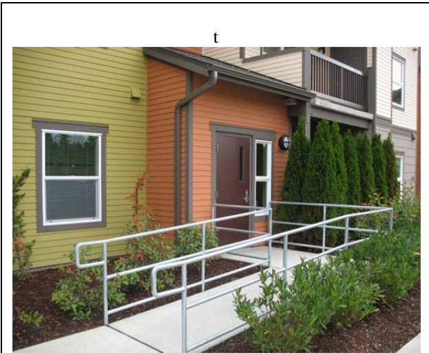
ADA egress from north(west) stairwell
