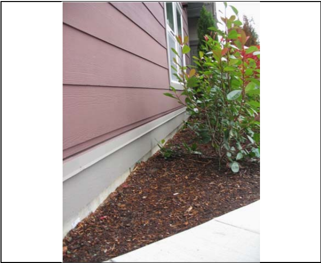
Foundation to wall transition and ground clearance
