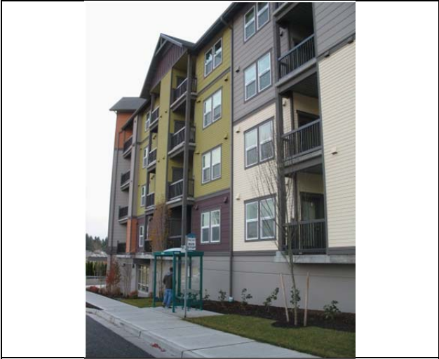
North elevation; 4 over 1, cement board and wood trim
